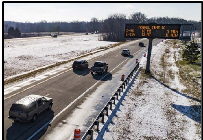
A dynamic message sign advertising expected travel times. Photo courtesy of MDOT.
