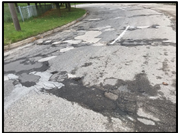
Poor pavement condition on Grand Rapids area street
