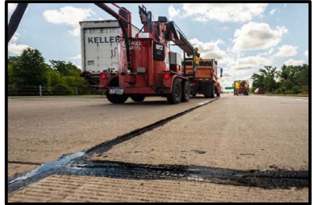
Crack sealing project; photo courtesy of MDOT
